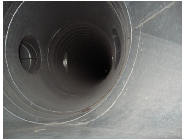
Air duct after cleaning
