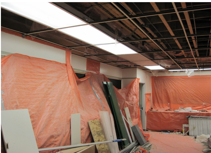
Measures must be taken to control the migration of dust and other contaminants
